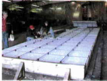
Workers affix steel reinforcing bar to a foam panel
